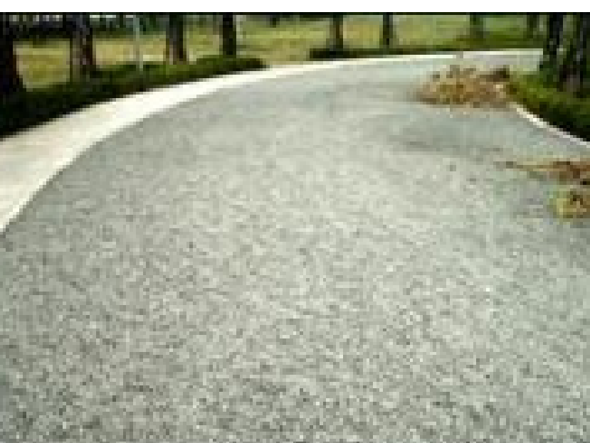
Pervious Concrete Paving
