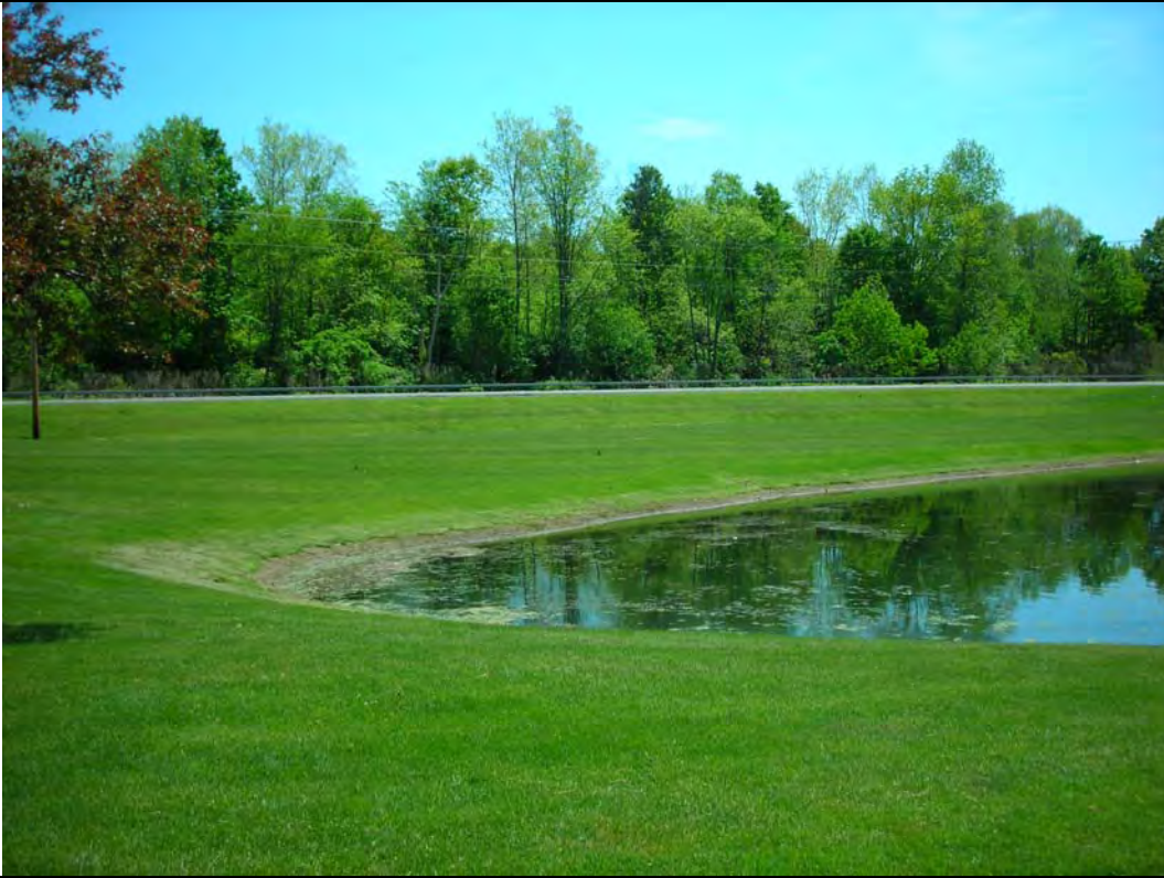
Photo #13: View east of Pond B with Route 22 in farground. The mowed area beyond the pond would be converted to an aquatic bench around the pond.
