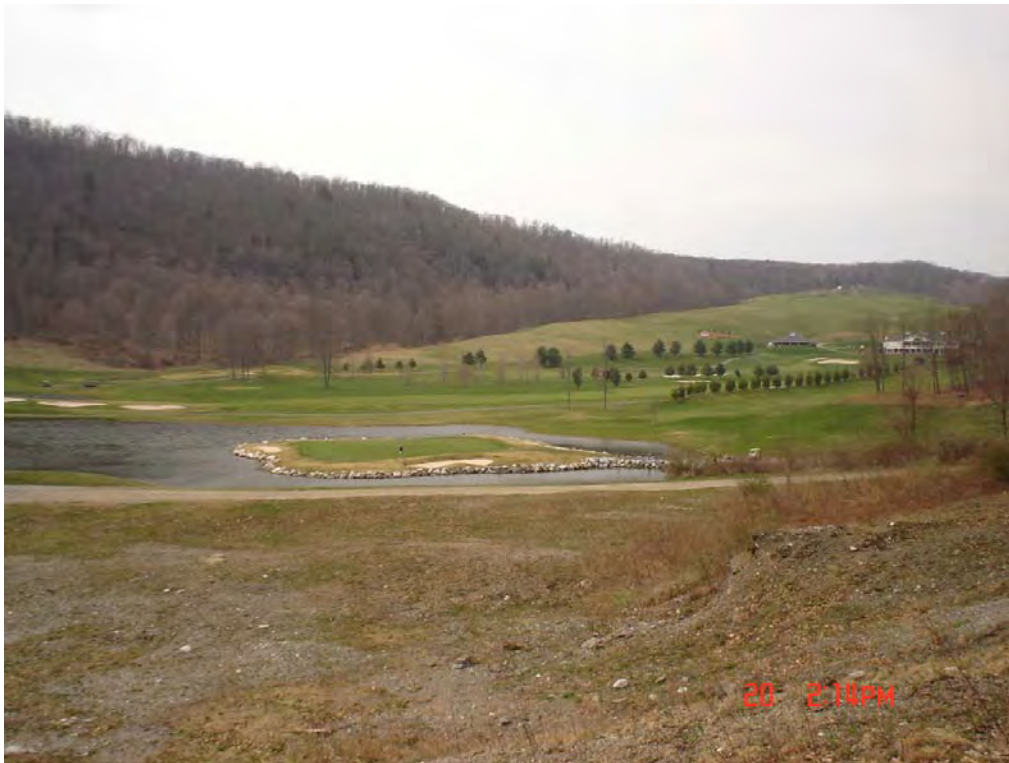
Photo #5: View to the northwest of island green illustrating pond, island green with riprap and remainder of pond edge. Island green will have marine seawall installed landward of riprap and ordinary high water mark, and after installation, riprap will be removed.
